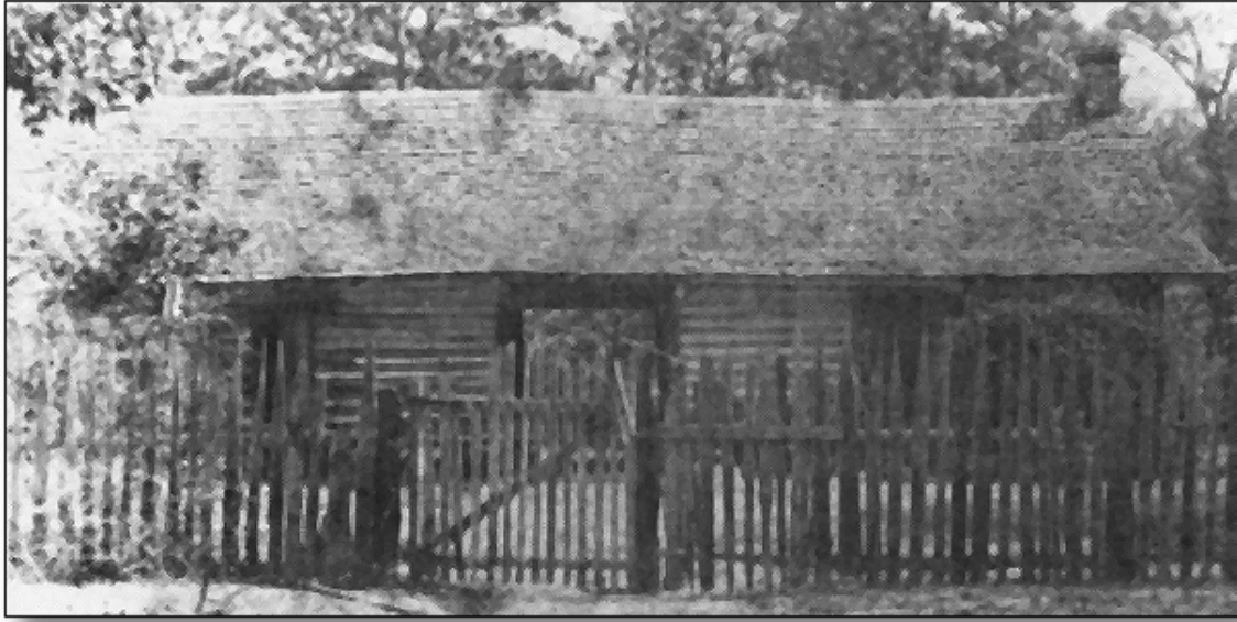
Homestead log cabin of Thomas Fain McMullen
