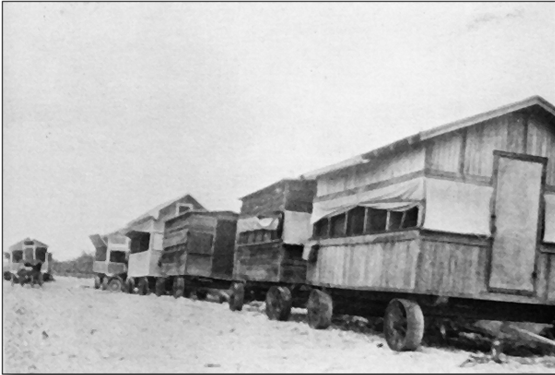
Rolling Bunkhouses— Work crew bunkhouses were pulled forward by oxen on the rough right-of-way an average of 150 feet a day. These were the first mobile homes in a state now numbering them in millions
