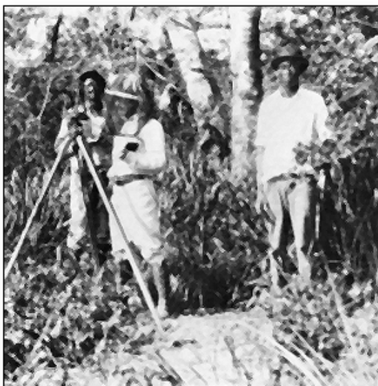
Tamiami Trail 1923. Surveyors—The first operation was to lay out the centerline of the road and then stakes were driven in the ground every 100 feet
