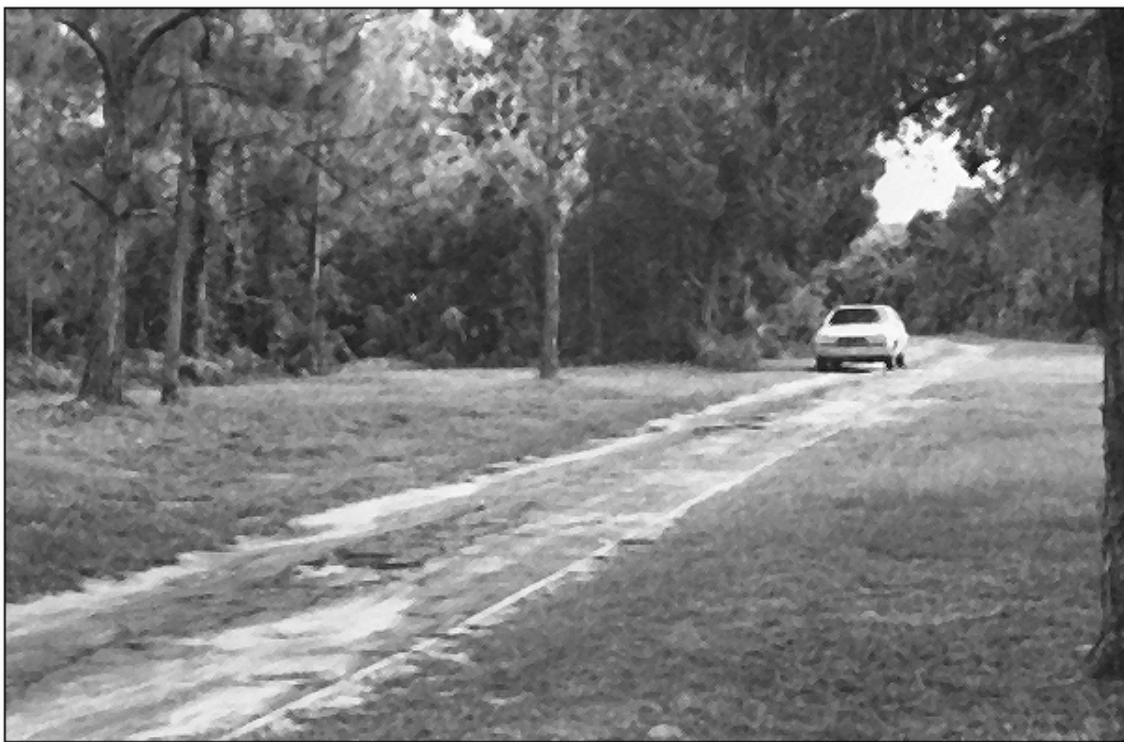
Tamiami Trail—One of the few remaining nine foot asphalt sections of the original Tamiami Trail between Sarasota and Venice at Eagle Point on Roberts Bay
